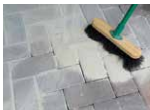
2. Brush into the joints
