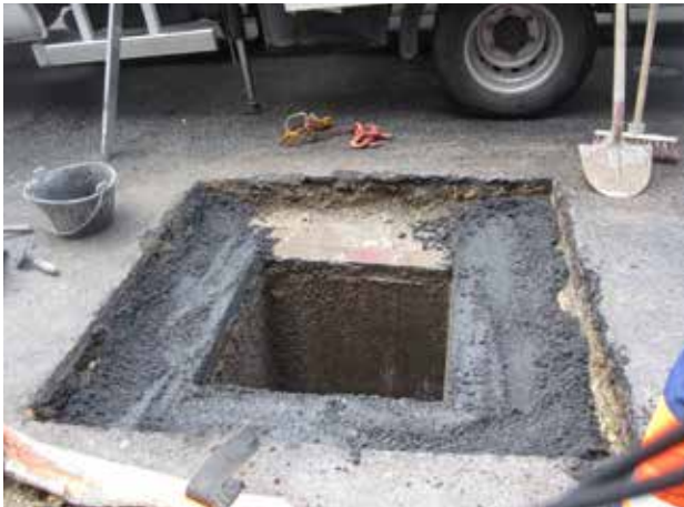
Placing Sika® FastFix-138 TT as a bedding mortar – mixed to a semi-dry consistency. Adjusting the final level of the manhole frame.
