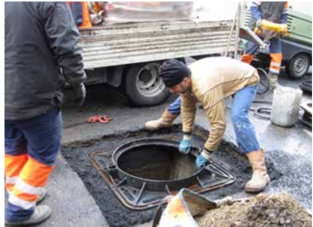
Placing Sika® FastFix-138 TT as a bedding mortar – mixed to a semi-dry consistency. Adjusting the final level of the manhole frame.
