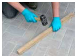
3. Compact well into the joints using a suitable Wacker-Plate, or simply use a wooden level and hammer.
