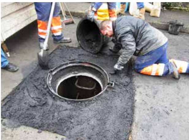
Pouring Sika® FastFix-138 TT to grout the manhole frame in position – mixed to a pourable consistency.
