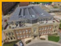
SINGLE PLY ROOFING
