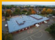
LIQUID APPLIED ROOFING
