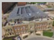
SINGLE PLY ROOFING
