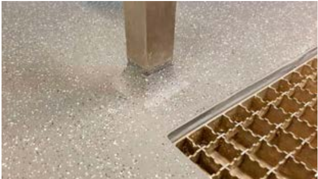
Kitchen and wetrooms
