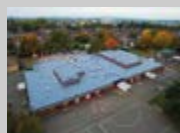
LIQUID APPLIED ROOFING
