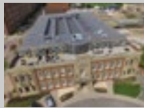
SINGLE PLY ROOFING
