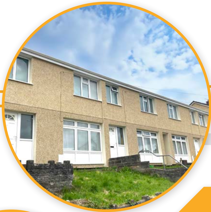
SWANSEA COUNCIL Refurbishment
